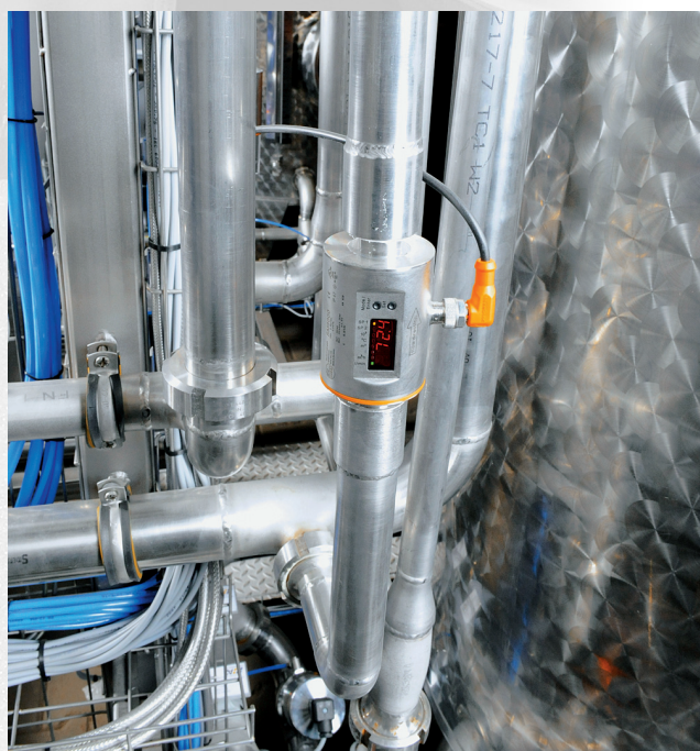
Volumetric flow sensor for the detection of the water quantity in a filtration system.
